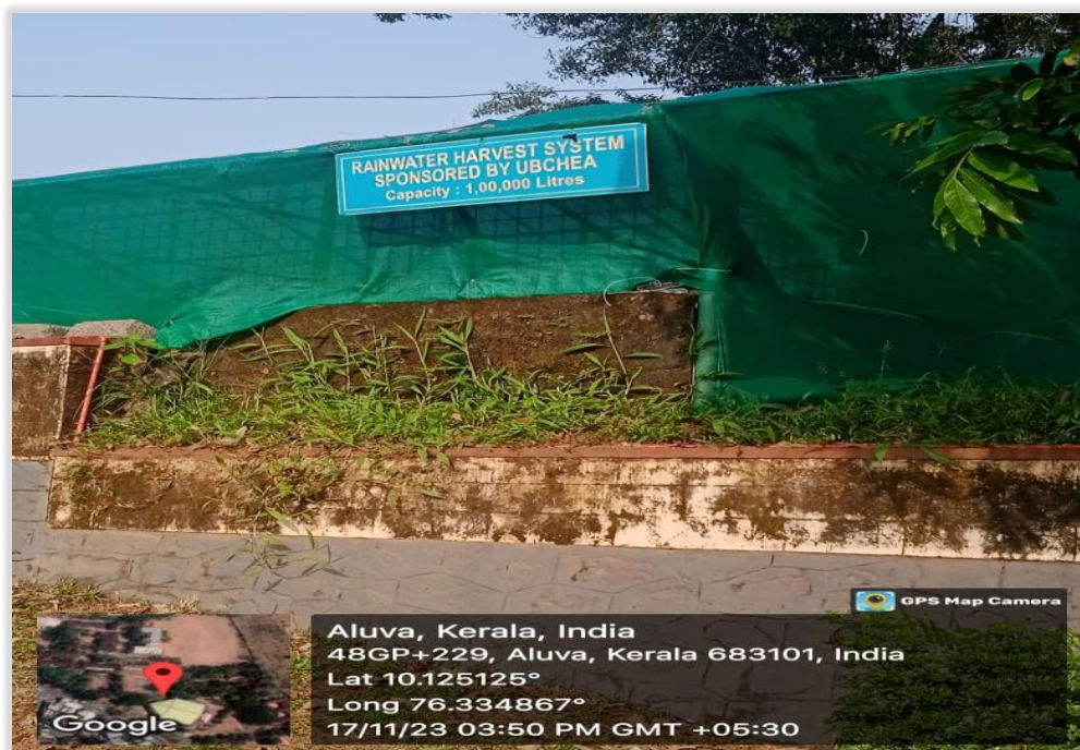
Figure 10 : Rain Water Harvesting System
