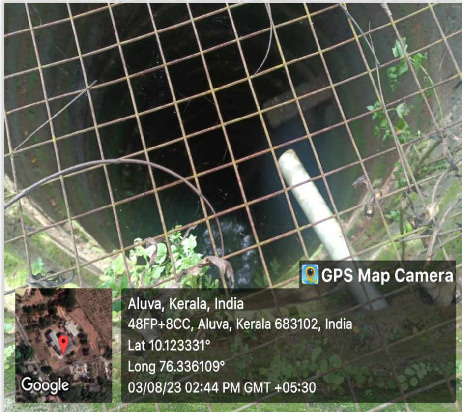
Figure 11 : Rain Water Recharge to Wells
